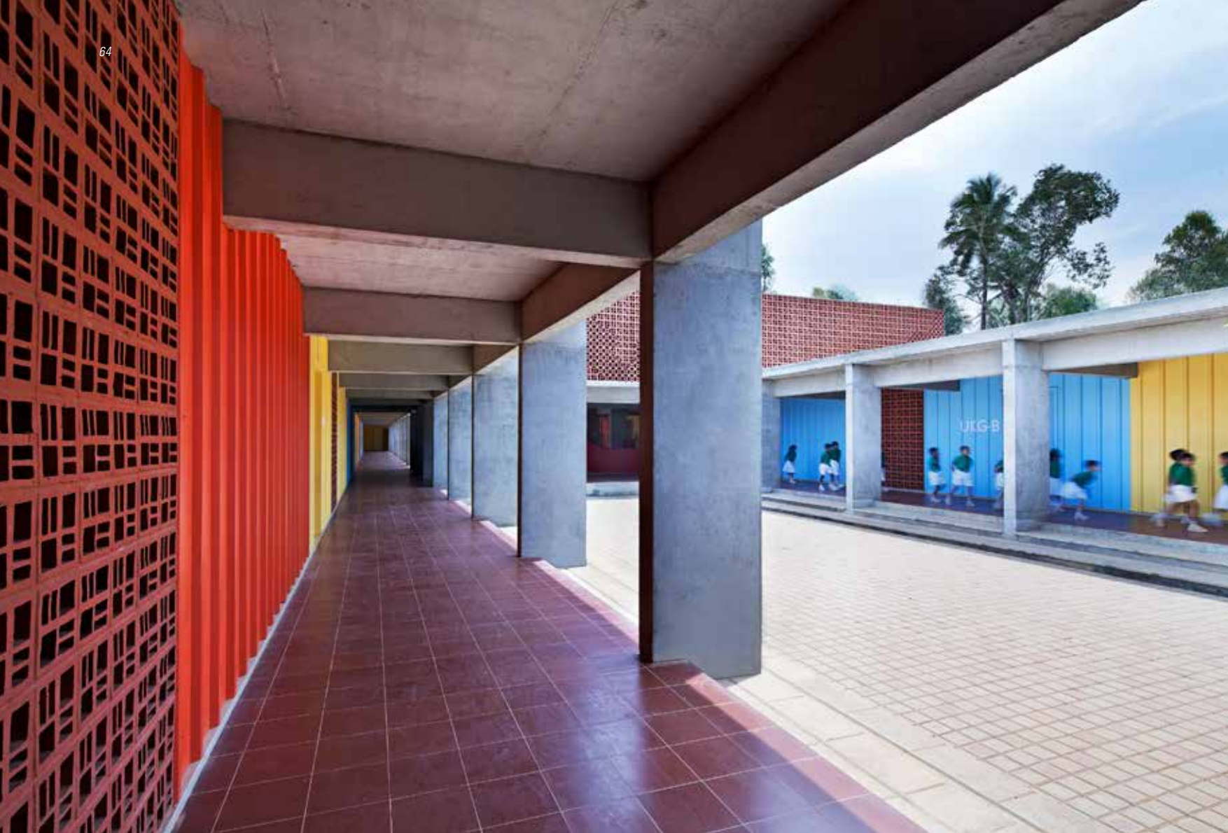
The 8ft wide single-loaded corridor with adjoining classes all around, effortlessly accommodates students, while offering an unobstructed view of the courtyard, drawing them into those spaces.
